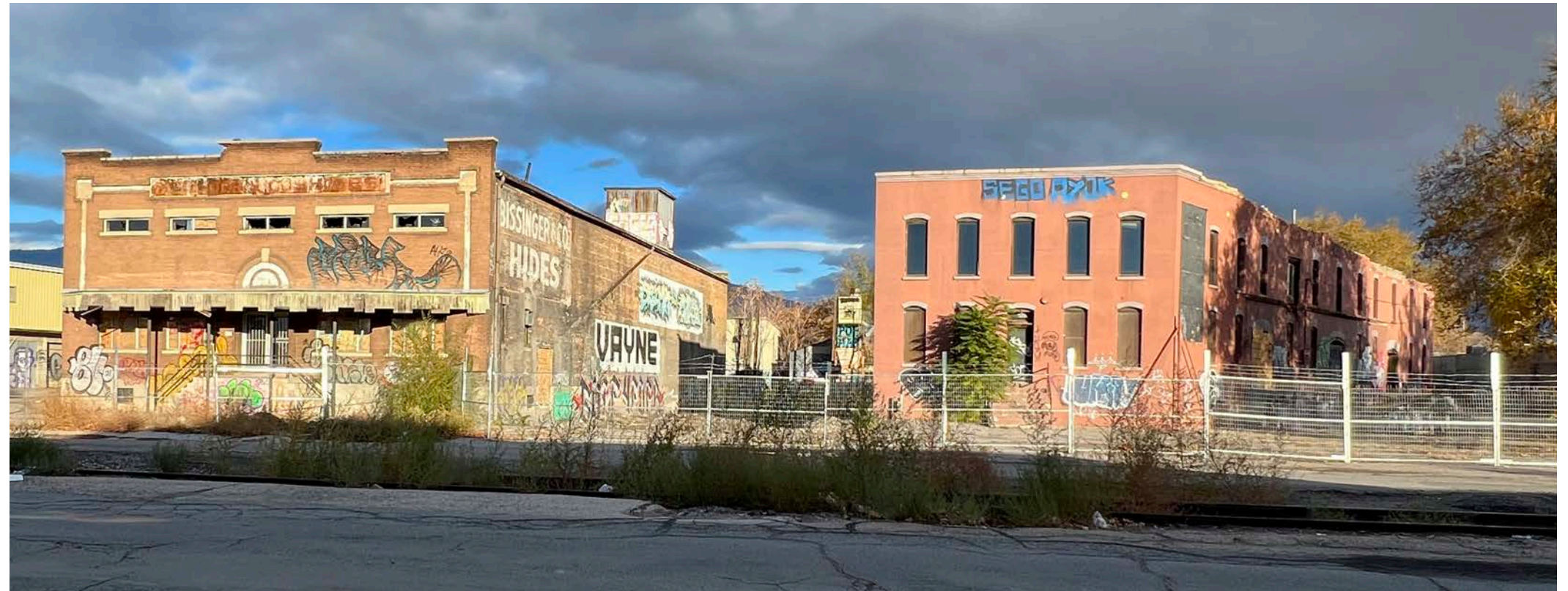
Existing Pickle and Hide buildings facing 400 West
