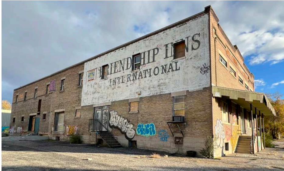
Northern facade of existing Hide building
