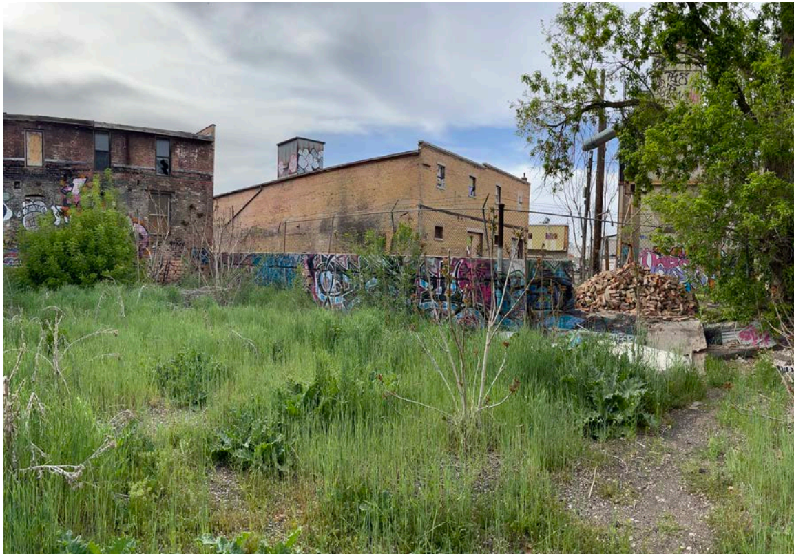
Eastern rear of site
